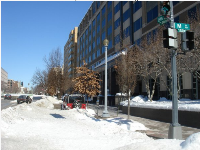
Above: NEA Headquarters 16 th and M, Washington, DC
